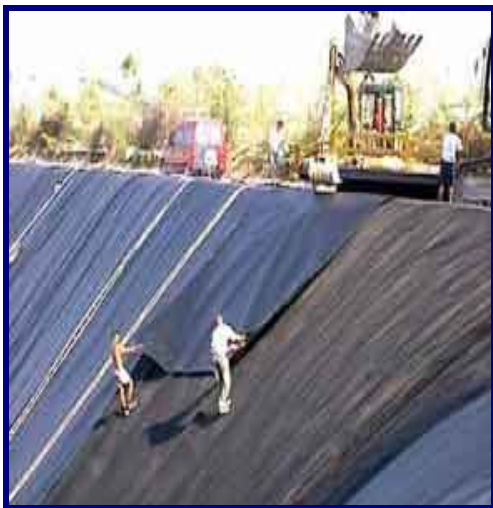
Deploying geo-composite over membrane liner sys- tem in landfill
