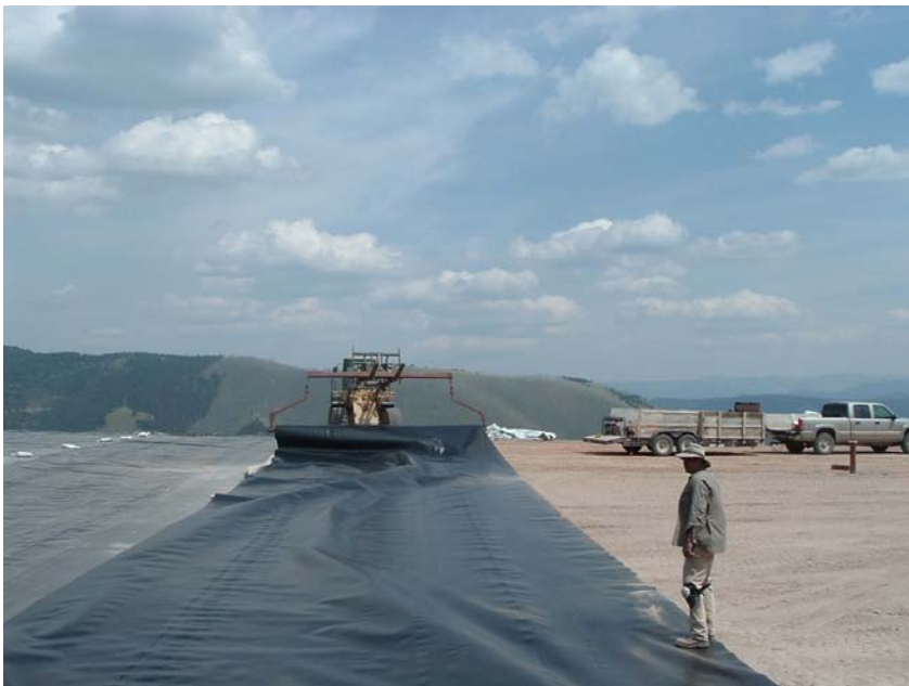
ARCO Mine, Phillipsburg MT
